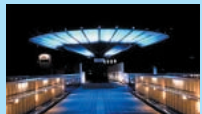
LED illumination systems installed in Hama-Otsu Sky Cross (promenade)
